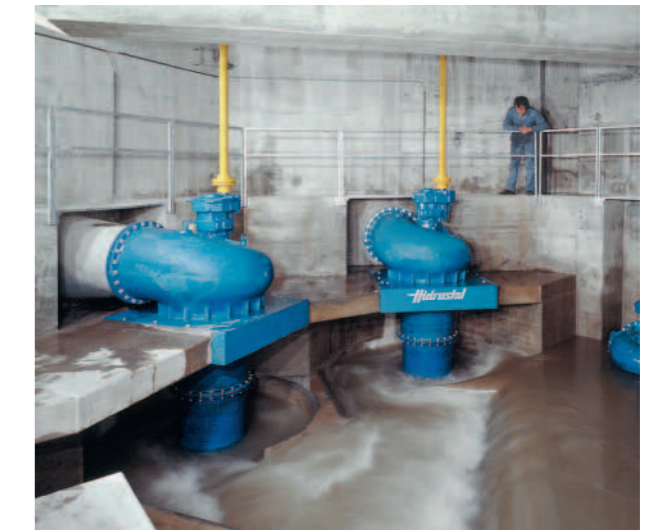
Sewage lift station with vertical installation and the PREROSTAL® flow regulating system.
